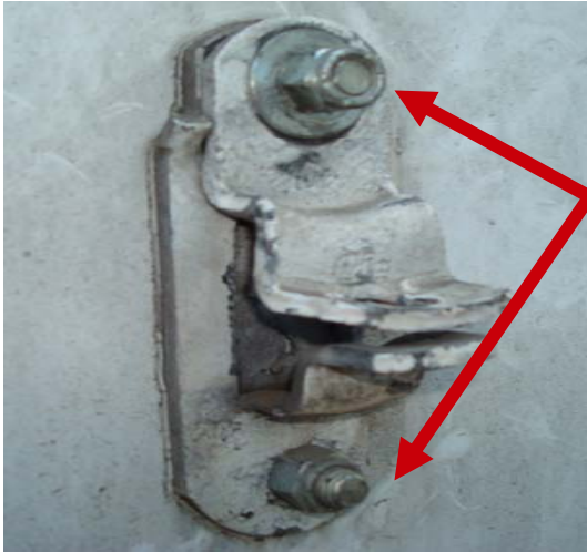
Different Bolts / Loosen Hasp
